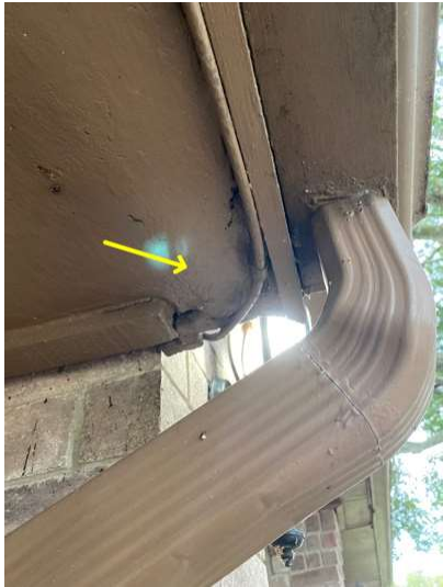
Wood deterioration
