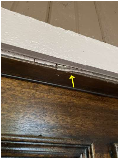
Caulking deterioration
