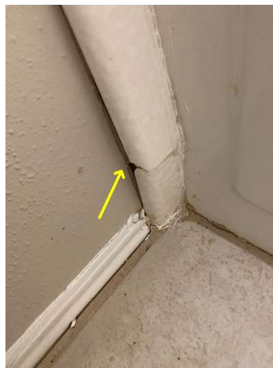
Damaged / pulling up - bathroom #1
