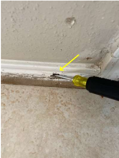
Wood deterioration - baseboard by back door
