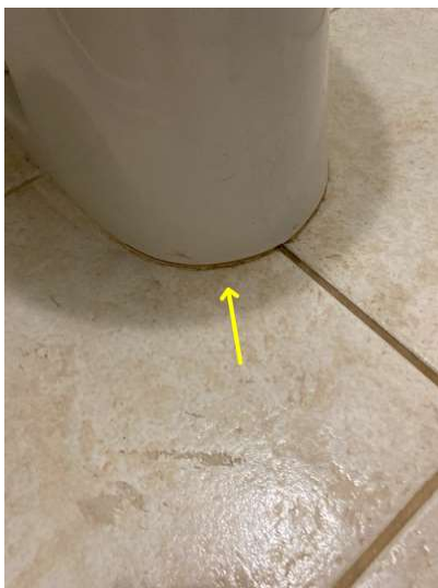
Caulking deterioration
