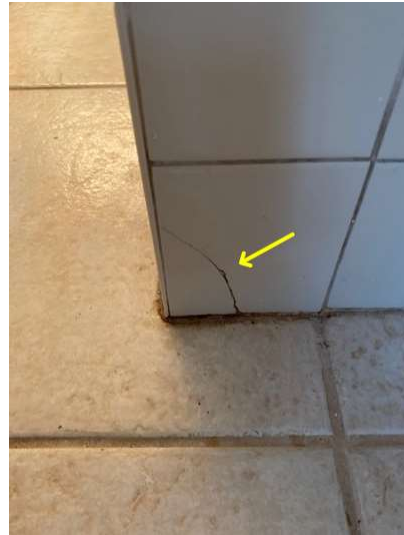
Cracked tile - bathroom #2
