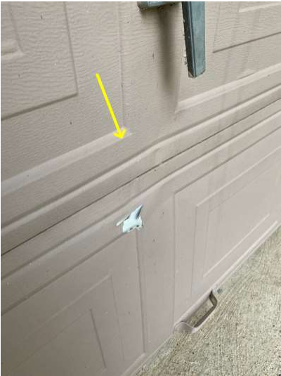
Dented and paint peeling - garage door
