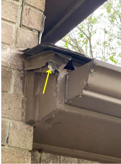
Damaged drip flashing
