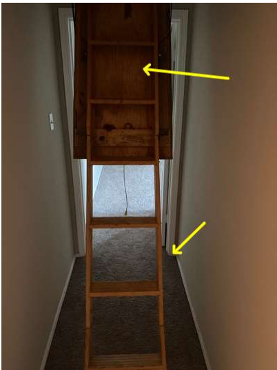
Loosely attached ladder and no insulation
