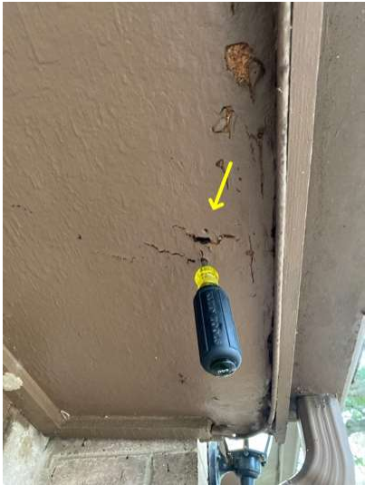
Wood deterioration
