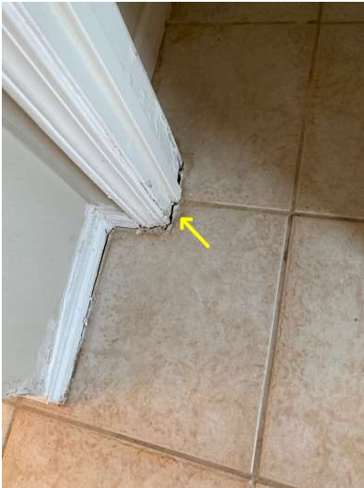
Caulking separation - Bathroom #2
