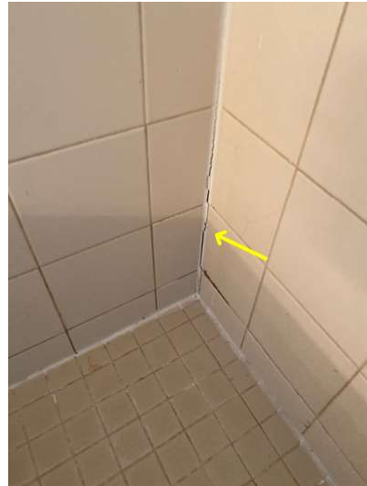
Caulking deterioration - bathroom #2
