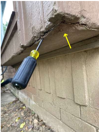
Wood deterioration
