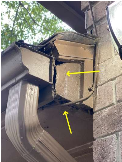
Wood deterioration
