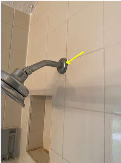
Loosely attached - bathroom #2
