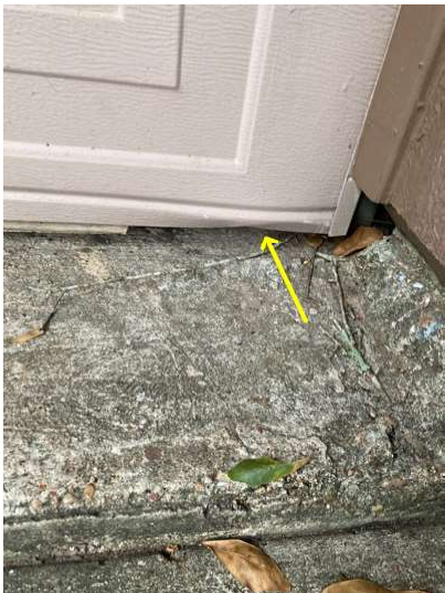
Damaged weather stripping
