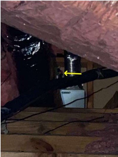
Exposed wires
