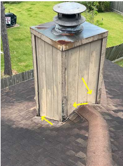
Wood deterioration
