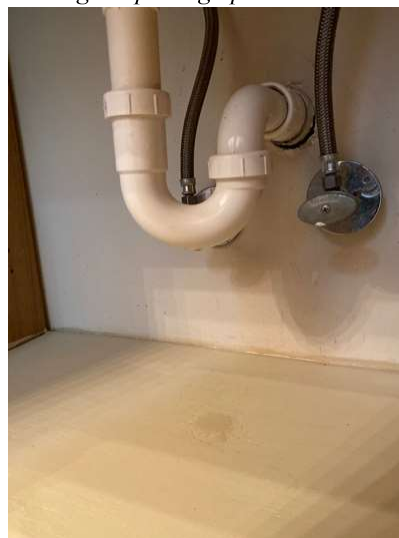
Water leak - bathroom #2
