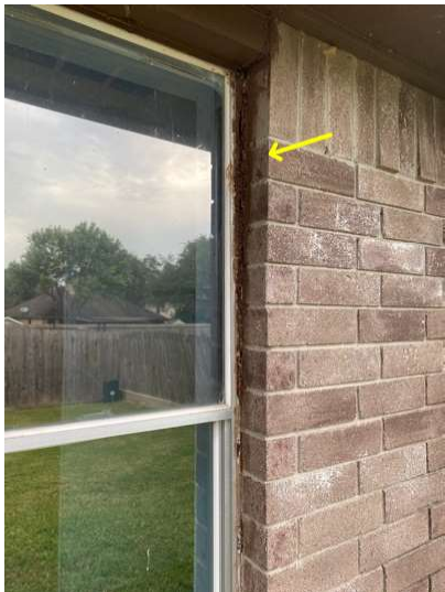
Caulking deterioration
